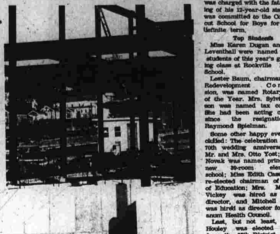
Rockville seen through girders of new court house.
